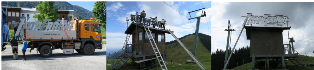
Figure 6: Installing Art Position 10 (Photos: Gerhard Pilgram)
